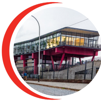
New Westbury Transformation Development Centre
