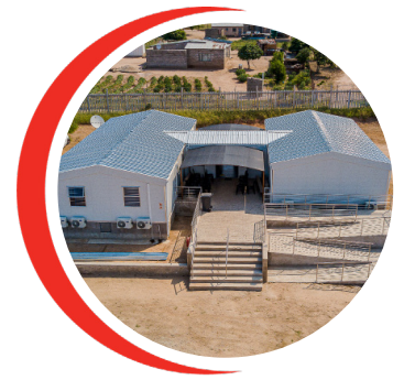
Upgrades to Makoko Clinic
